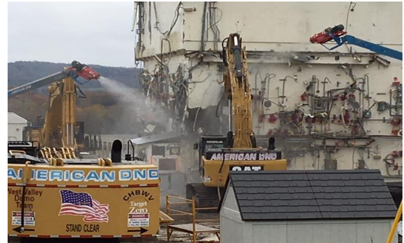
Demolition of WVDP Vitrification Facility
