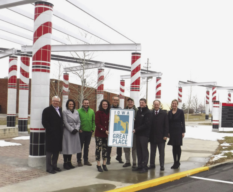
The Waukee Railroad Pergola project received the Iowa Great Places designation from the Iowa Department of Cultural Affairs for its success in facilitating creative placemaking. The 350-foot-long installation is a trailhead gateway and the centerpiece of a regional plan to unify and develop the 89-mile rural Racoon River Valley Trail Corridor as a nationally recognized visitor destination.
