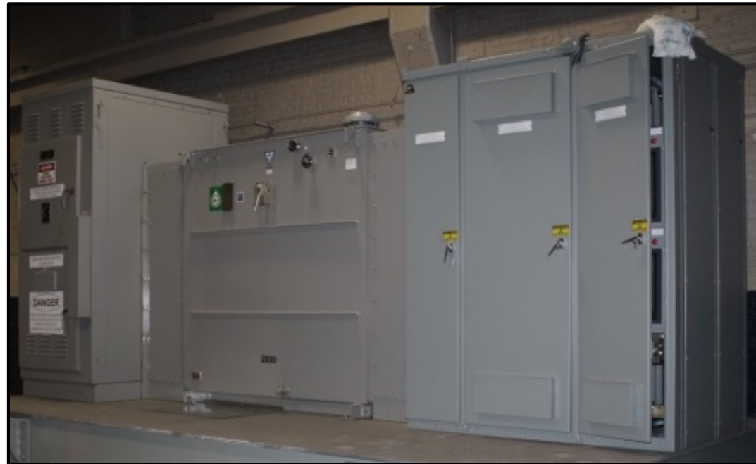
NEW SUBSTATION REQUIRED FOR POWER CAPACITY
