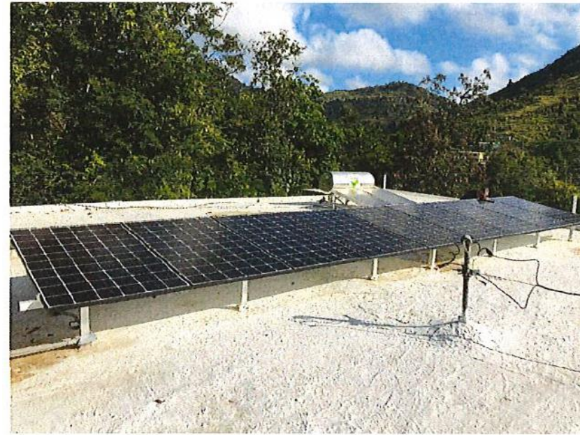
A PV and battery storage system installed in Puerto Rico as part of this proj
