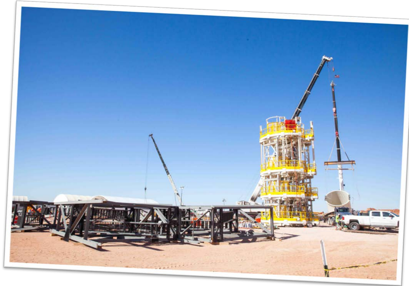
Utility shaft headframe and Galloway work platform.
