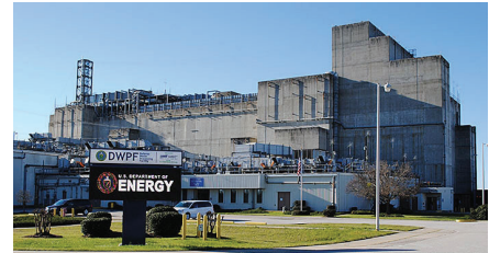
FIGURE 15: The Savannah River Site defense waste processing facility. Photo courtesy of U.S. Department of Energy.
