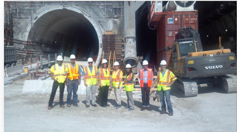
Port of Miami Tunnel
