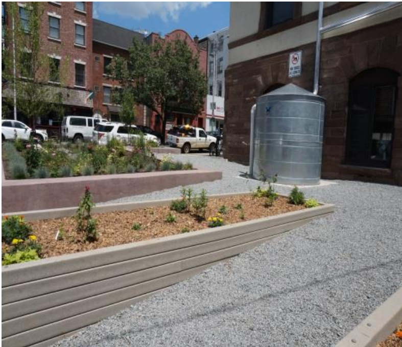
Green Infrastructure – Cistern / Rain Garden
